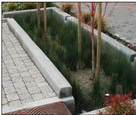
Figure 7 – Typical planter box (Source: Philadelphia Water Department, 2014)
