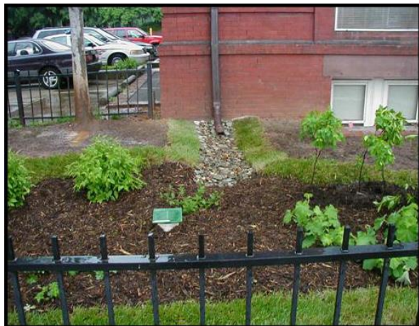
Figure 4 – Typical downspout disconnection configuration (Source: LID Center, 2005)
