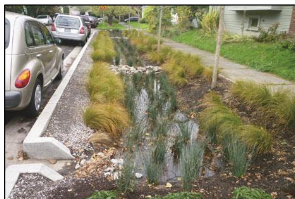
Figure 8 – Typical urban bioswale (Source: American Forests, 2012)
